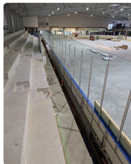
New spectator glass installed along the grandstand side.
