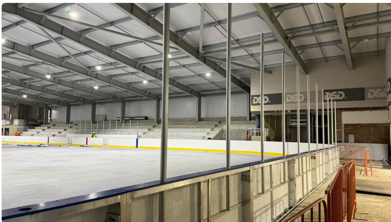
Looking down the pad from the sideline, with the grandstand beyond.
